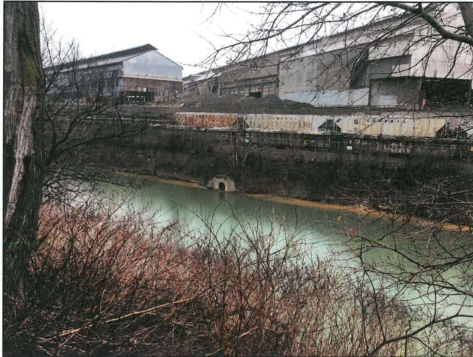
Photograph 1 – View of existing concrete headwall of 48-inch diameter culvert conveying Trib 64495 to Turtle Creek. The enclosed stream culvert is buried nearly 20 feet below existing ground surface. View is facing north.
